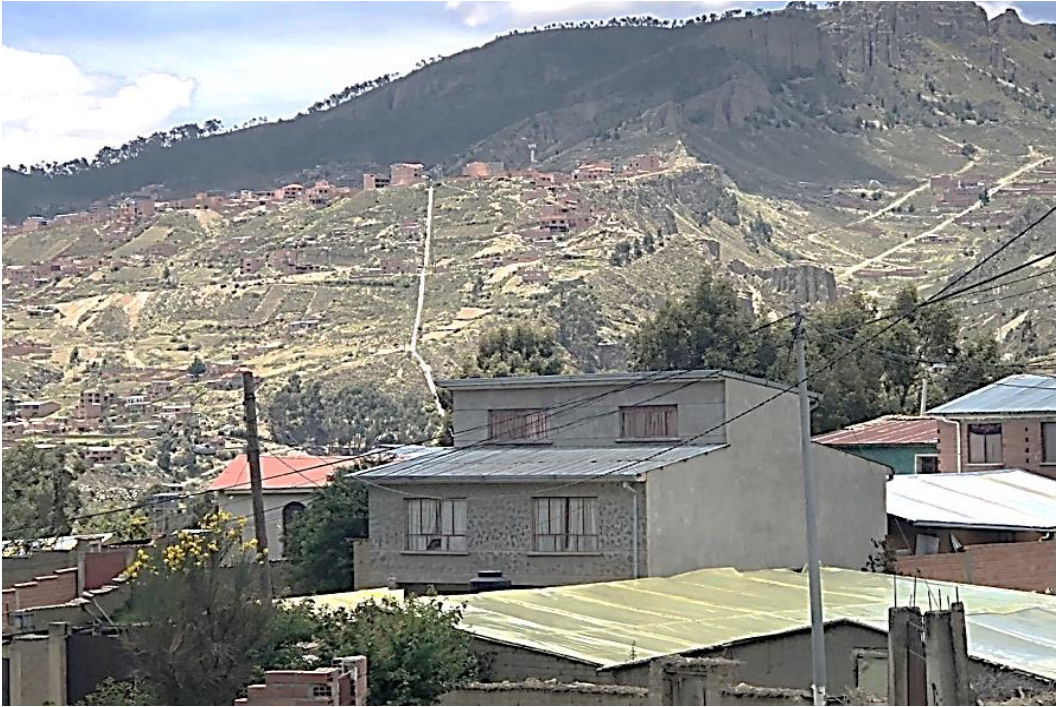
Picture 1. La Paz (municipality). Water pipe channeled from the Hampaturi dam (taken from Chinchaya) Photo: E. Torrico, 2018
